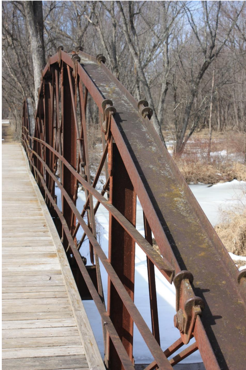
Single rolled beam for the top chord
