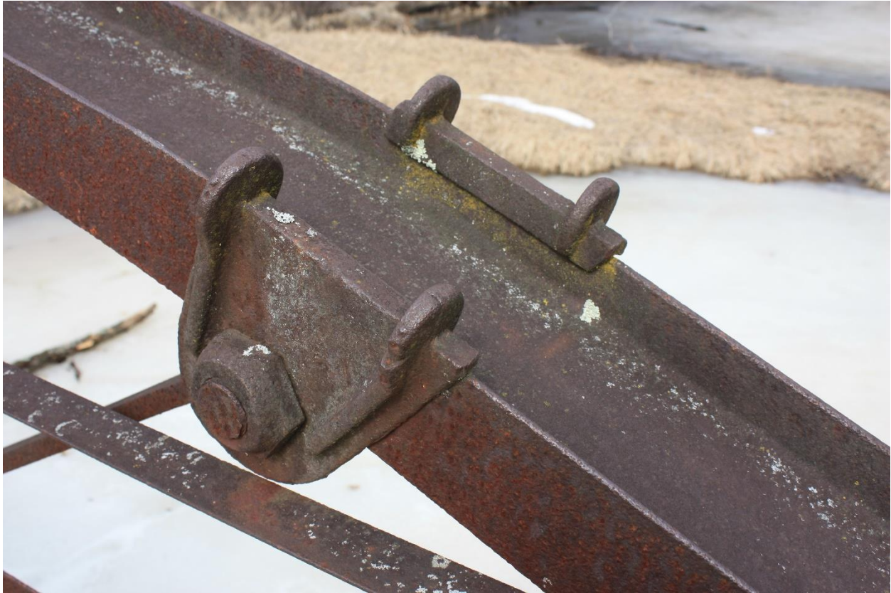
Clips gripping the top chord
