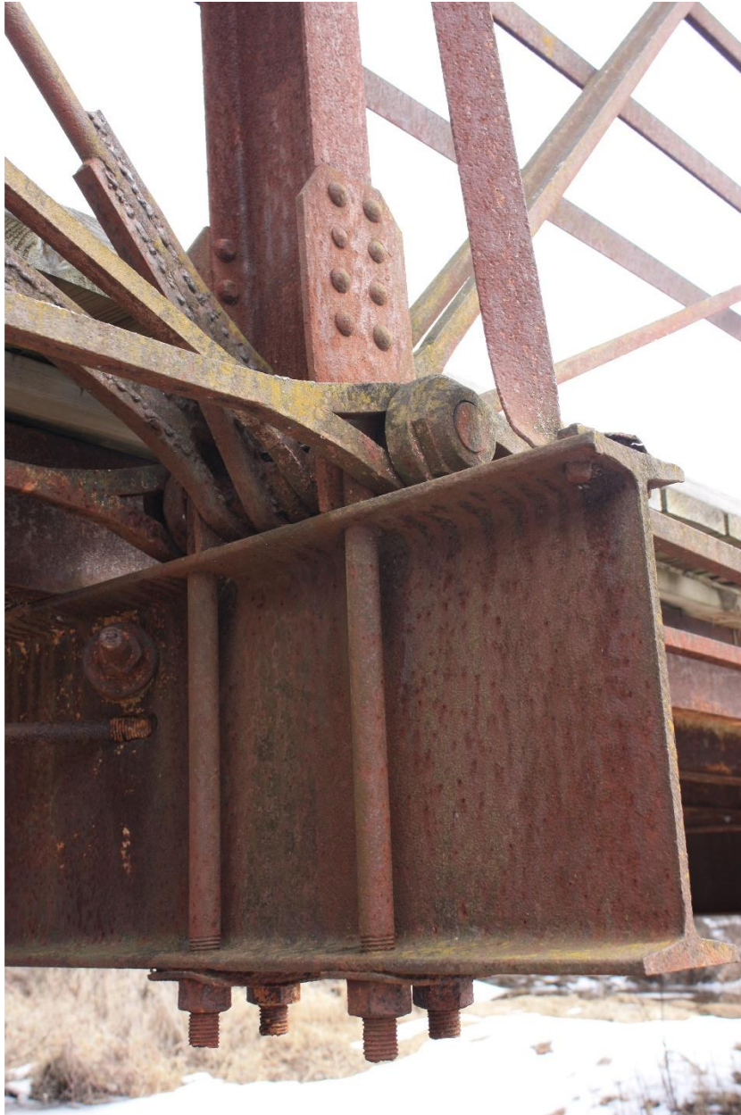
U-bolt connections to the deck beam
