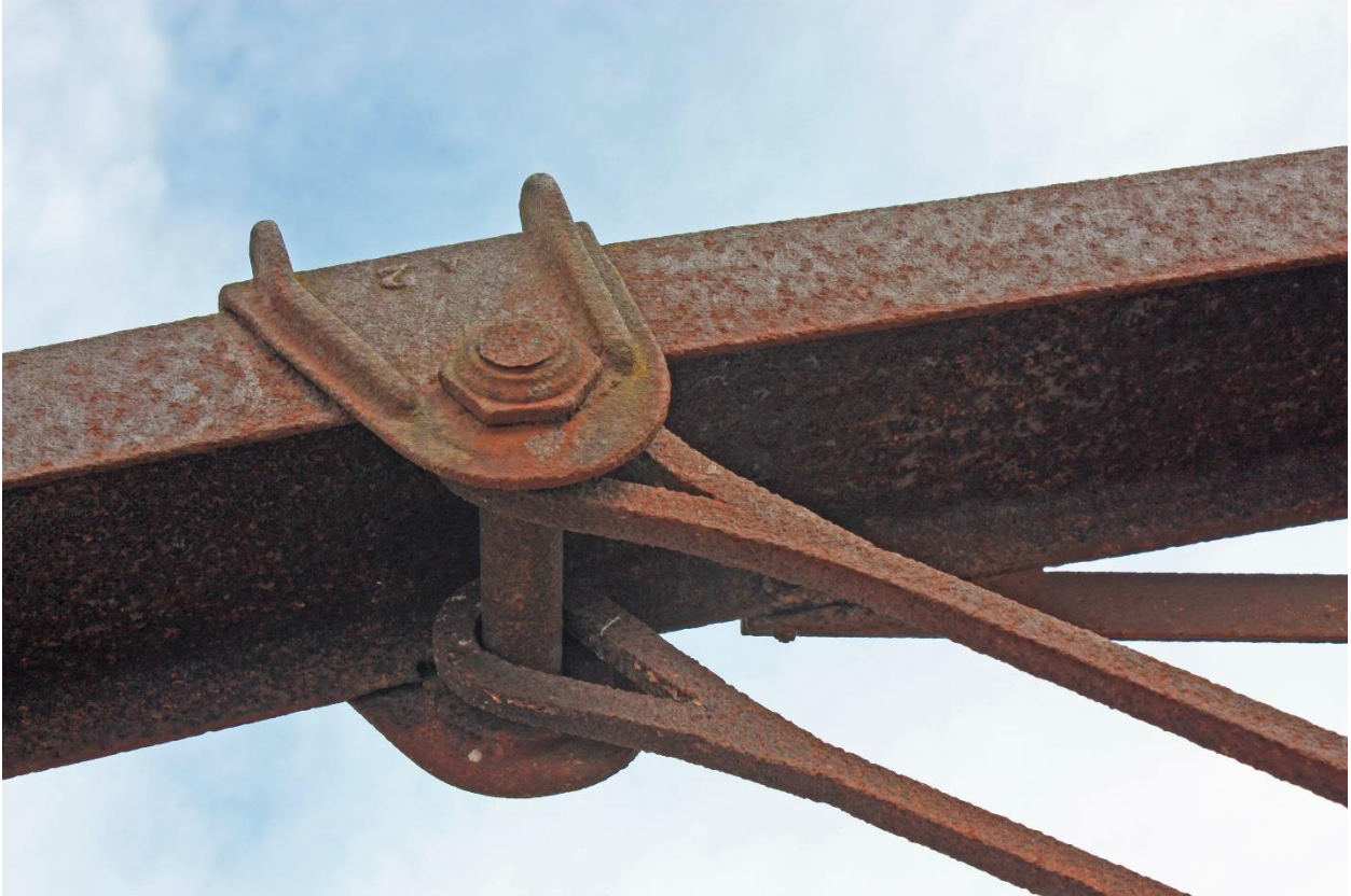
Underside of a clip attaching diagonal supports
